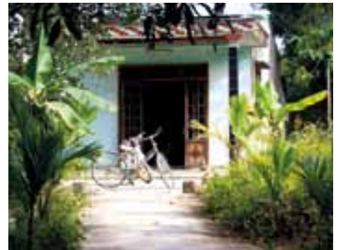
Flood-resilient housing, Vietnam – Chris Goldberg
