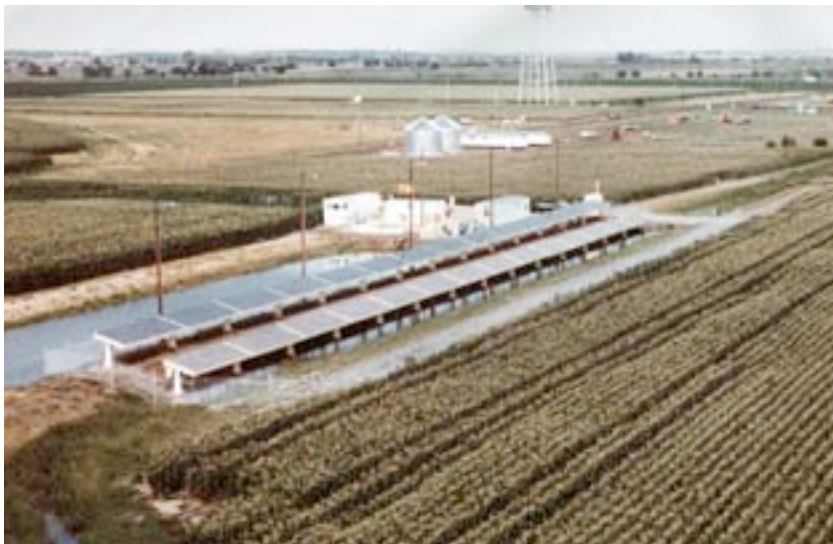
Figure 2: Solar Panels are grouped in large arrays in order to collect more sunlight and produce more energy. These are placed along a cornfield. Source: NASA
