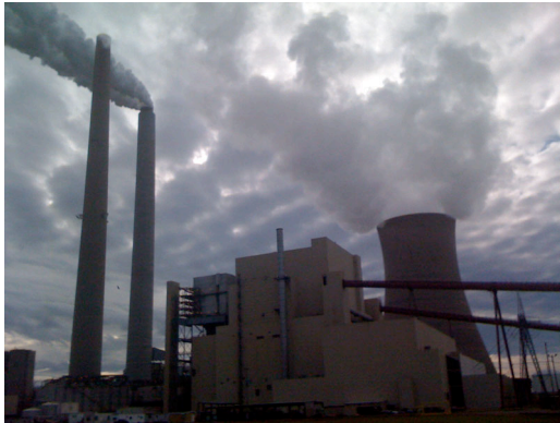
The Mountaineer Power Plant in West Virginia
